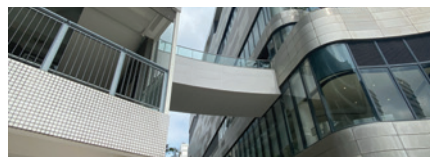
Completion of link bridge connecting R and C Block
